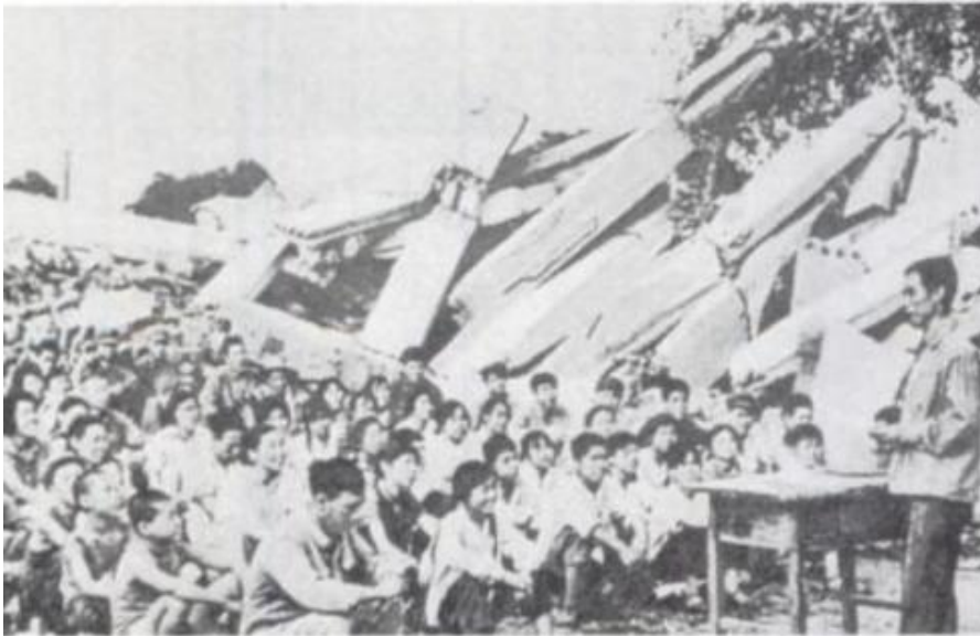
Collapse of precast buildings in Tangshan, China 1976
