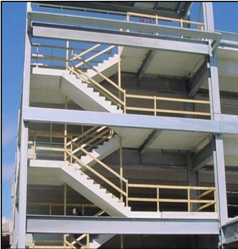
Precast concrete Stairs
