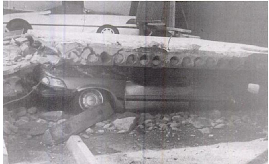
Collapse of Precast Concrete Hollow Core Floor; 1994 Northridge Earthquake, California
