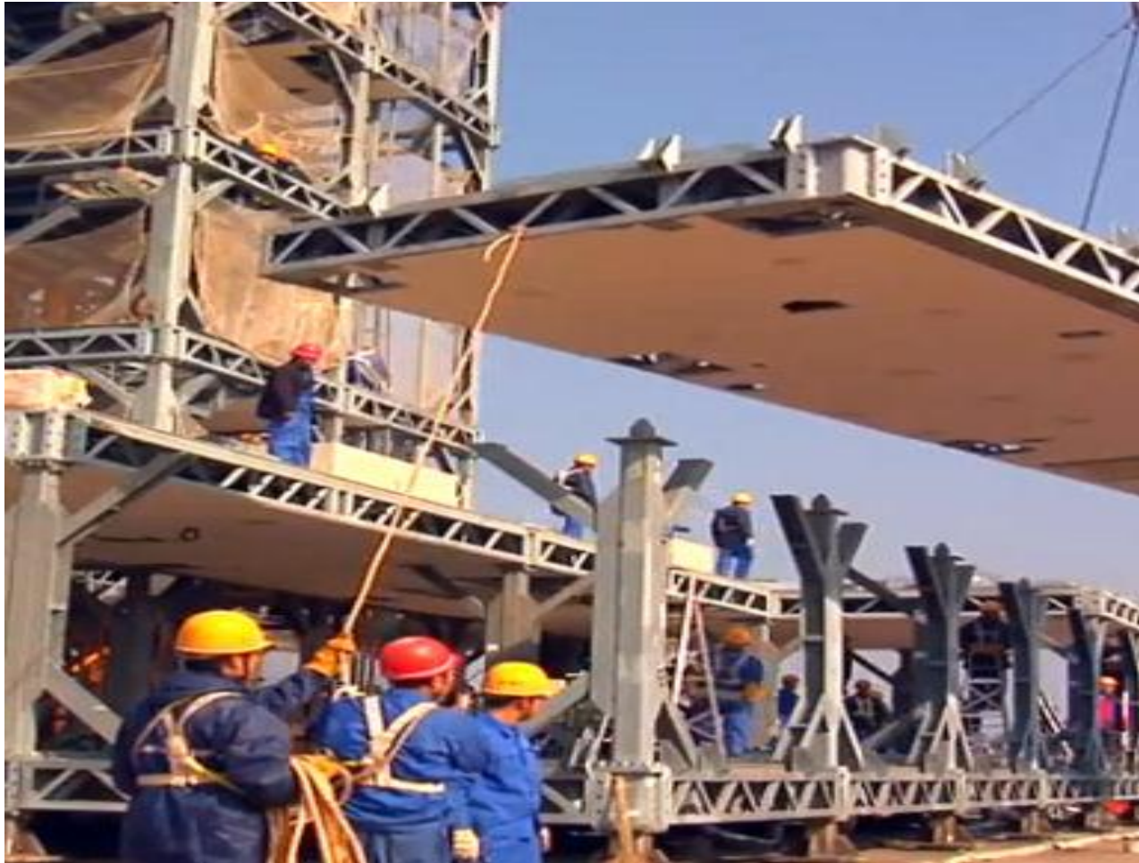
Installation of a Slab
