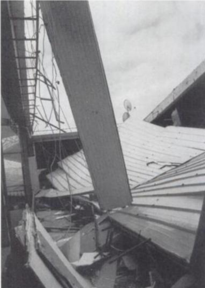
Failure of Flexible light-gauge metal diaphragm; 1999 Kocaeli Earthquake, Turkey
