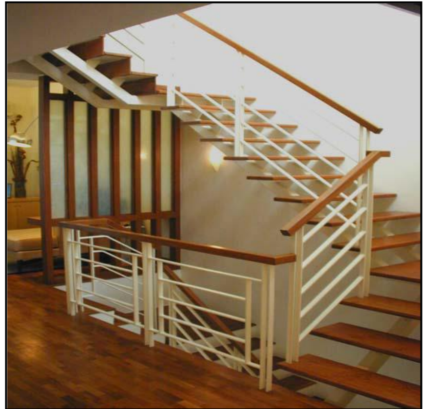
Steel plates supported on 2 steel beams
