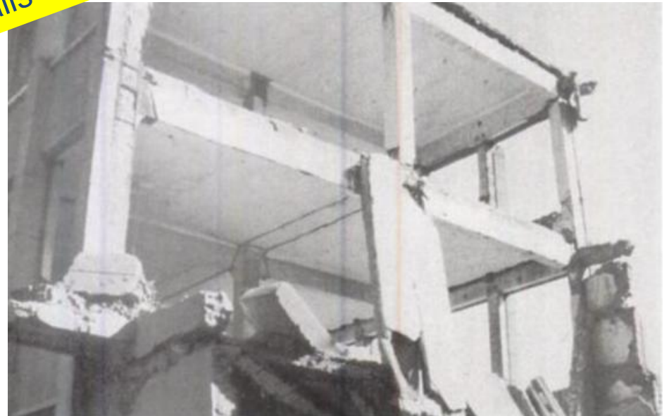
Failure of a poorly detailed beam-column connection (1976 Tangshan earthquake, China)
