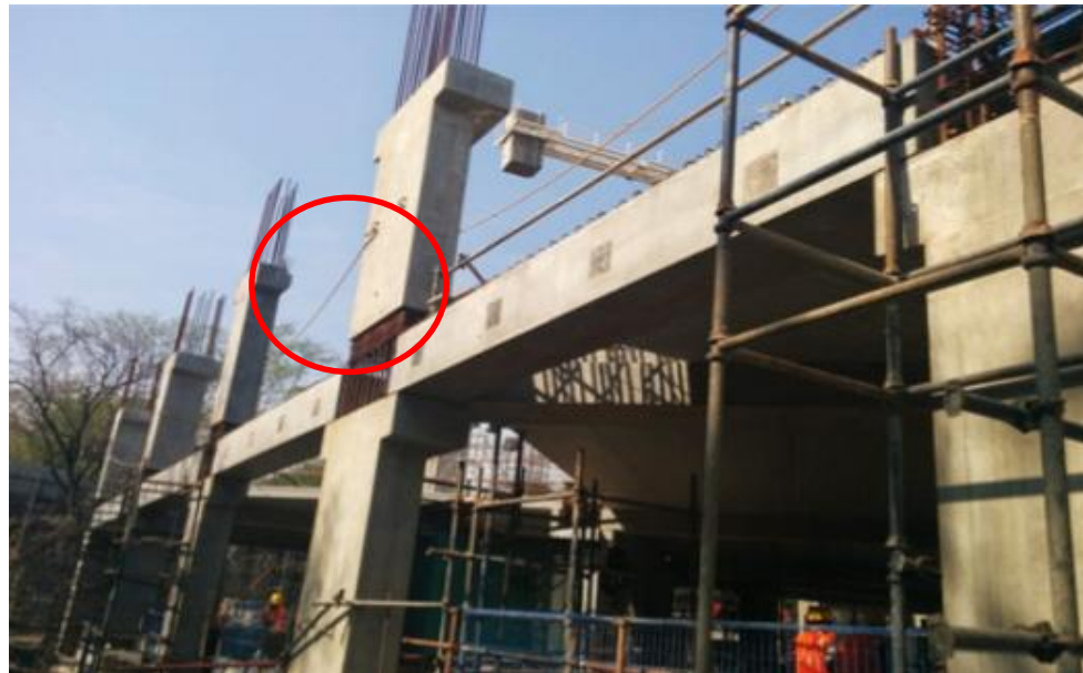
Peripheral Column-beam joint
