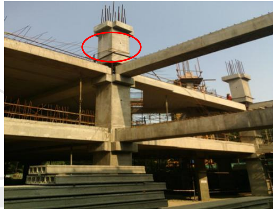
Interior Column-beam joint
