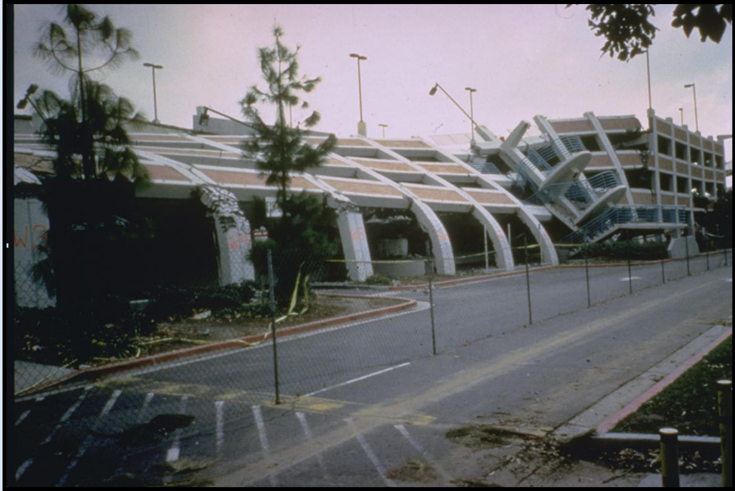
Precast parking structures
