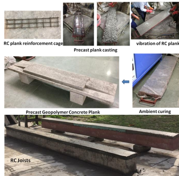
Fig. 1: Casting of RC Plank & Joist from Geopolymer Concrete
