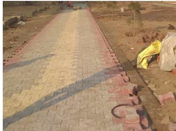
Fig. 4(b): Paver Block laying at Construction Technology Demonstration Park at CBRI
