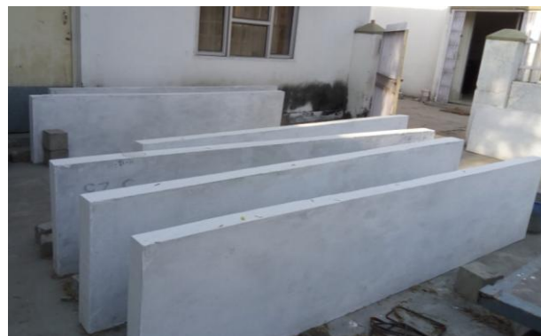
Fig. 4: Sandwich Panels Cast
