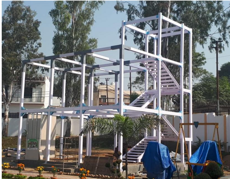
Fig. 3: Framed Structure of Dry Construction System for EWS Type House
