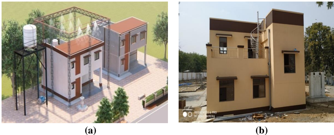
Fig. 1: Proposed Test Setup for Water Tightness Evaluation of Housing System
