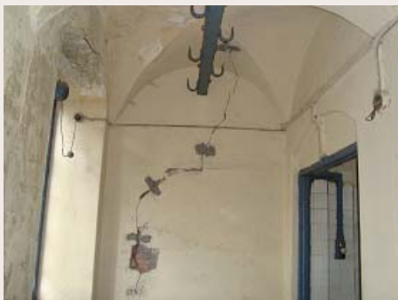
Photo 2 : Cracks in the Walls and Vault of Western gallery and dampness marks
