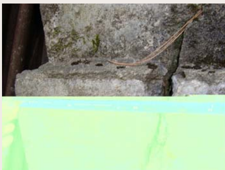
Photo 3 : Crack at foundation level on in the buttress wall North Side
