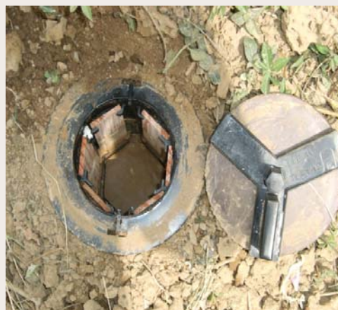
Photo 11: Internal view of an IGBS with wooden interceptors
