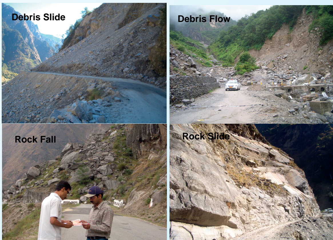
Fig. 1: Landslides of different types along Chamoli-Joshimath Road
