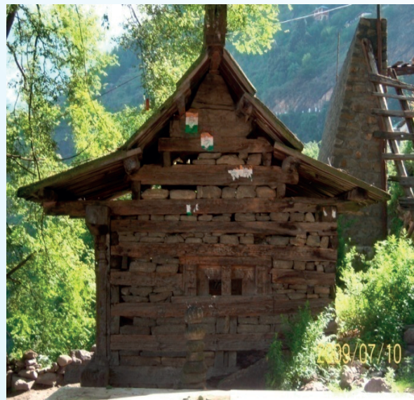
Typical building structures of Uttarakhand using Coarsed/un-coarsed Random Rubble masonry with wooden logs
