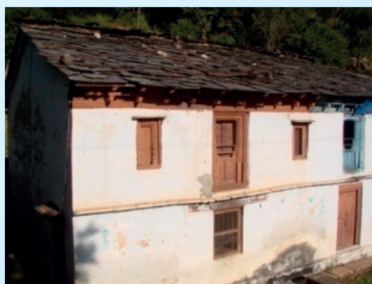
A Traditional double story house using Random Rubble masonry, wood and slates
