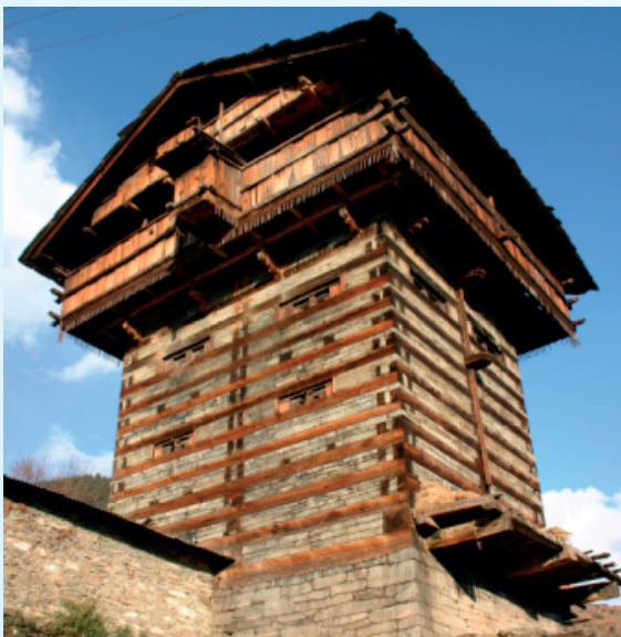
Typical building structures of Uttarakhand using Coarsed/un-coarsed Random Rubble masonry with wooden logs
