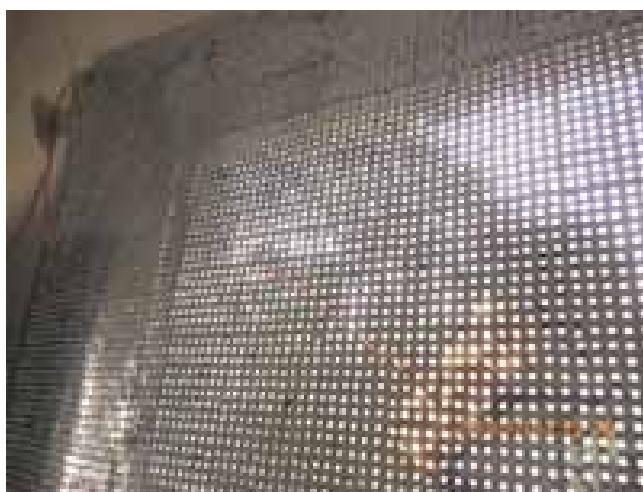
Fig.1: Perforated GI Sheet- 4 mm holes
