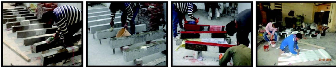
Fig.6 (a-d): Procedure for FRP application
