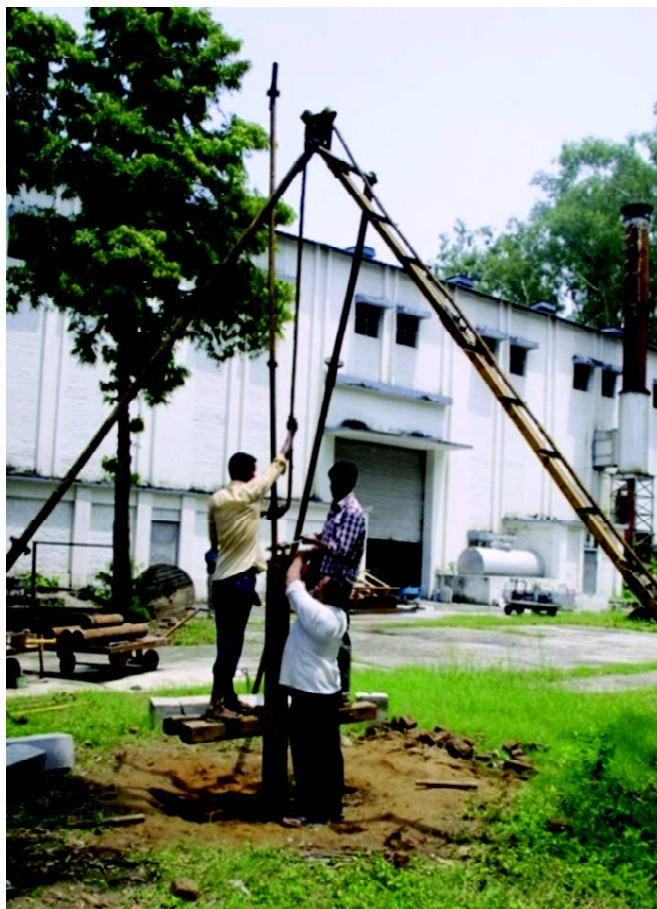
Drilling of Borehole in progress
