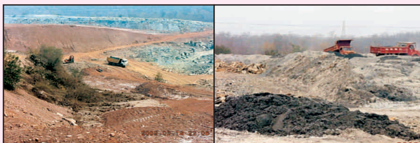
Construction of red mud pond utilizing Red Mud and Ash
