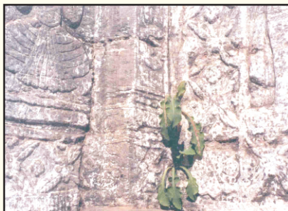
Fig.1: Initial stage for the deterioration of the cementitious materials
