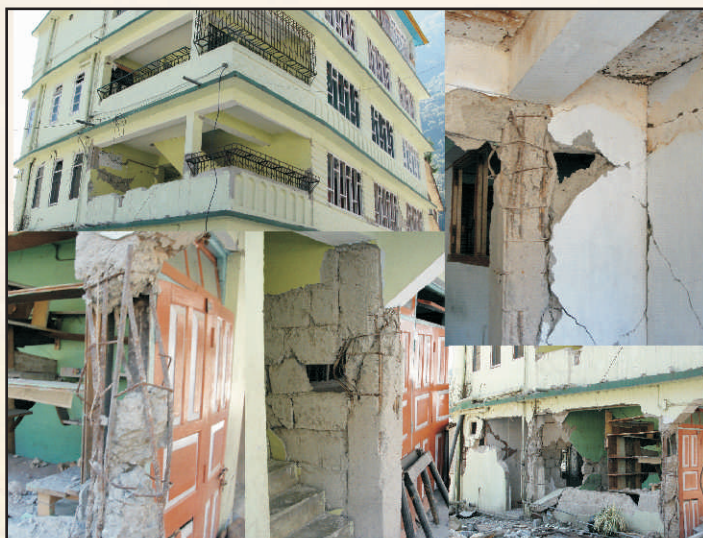
Fig. 4: Typical failure of RC buildings in Chungthang (Sikkim)
