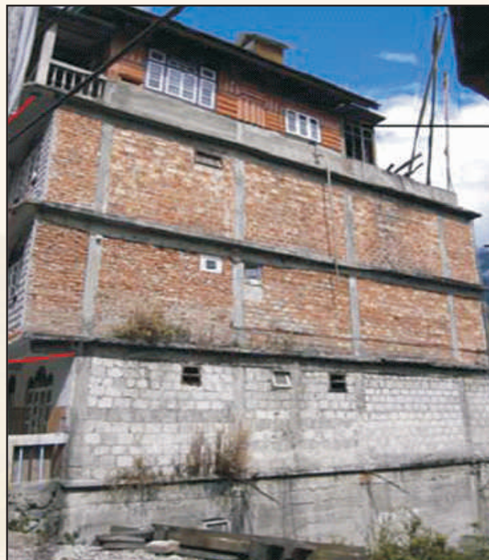
Fig. 5 : Typical hybrid infill RC construction in Lachung (Sikkim)
