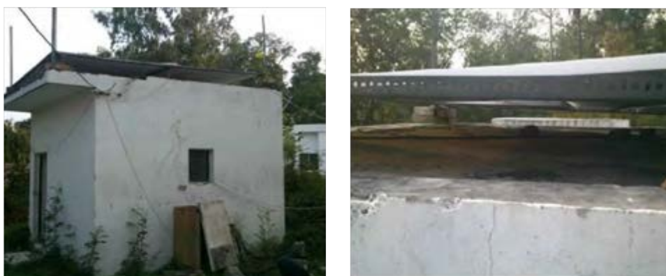
Fig. 1: (a) Experimental room with double deck roof (b) Close up view of DDR with air gap
