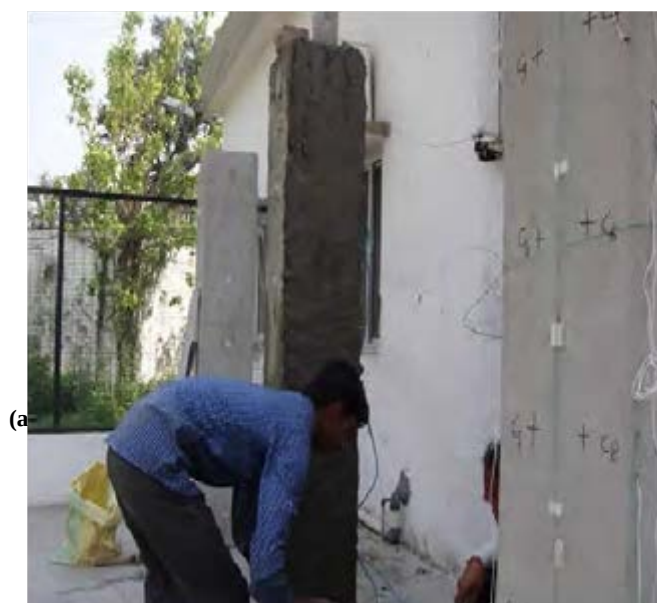
Fig. 1: Three RC columns for experimental CP application. Placement of conductive overlay on middle column (ICCP) in process
