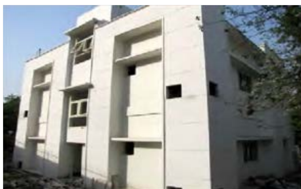
Fig. 2: Rear side (south-west facade) of the building with recessed openings and locating toilets and staircase for minimizing heat flux to rooms
