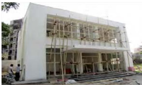
Fig. 1: Front (north) facade of the building with proposed tempered glass for glass cleaning robot
