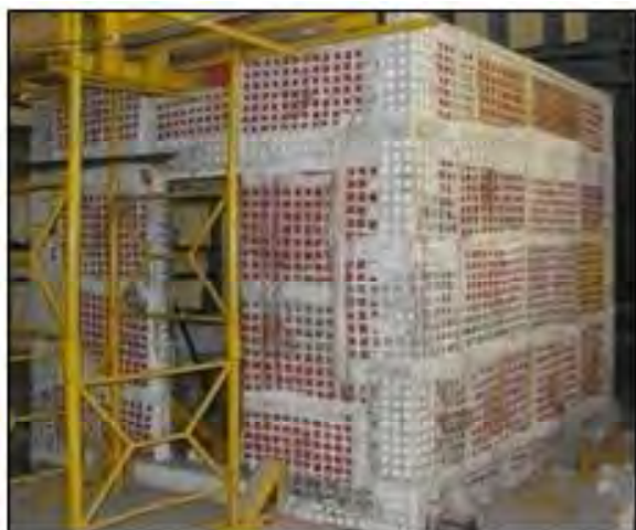
(c) Plastering and curing
