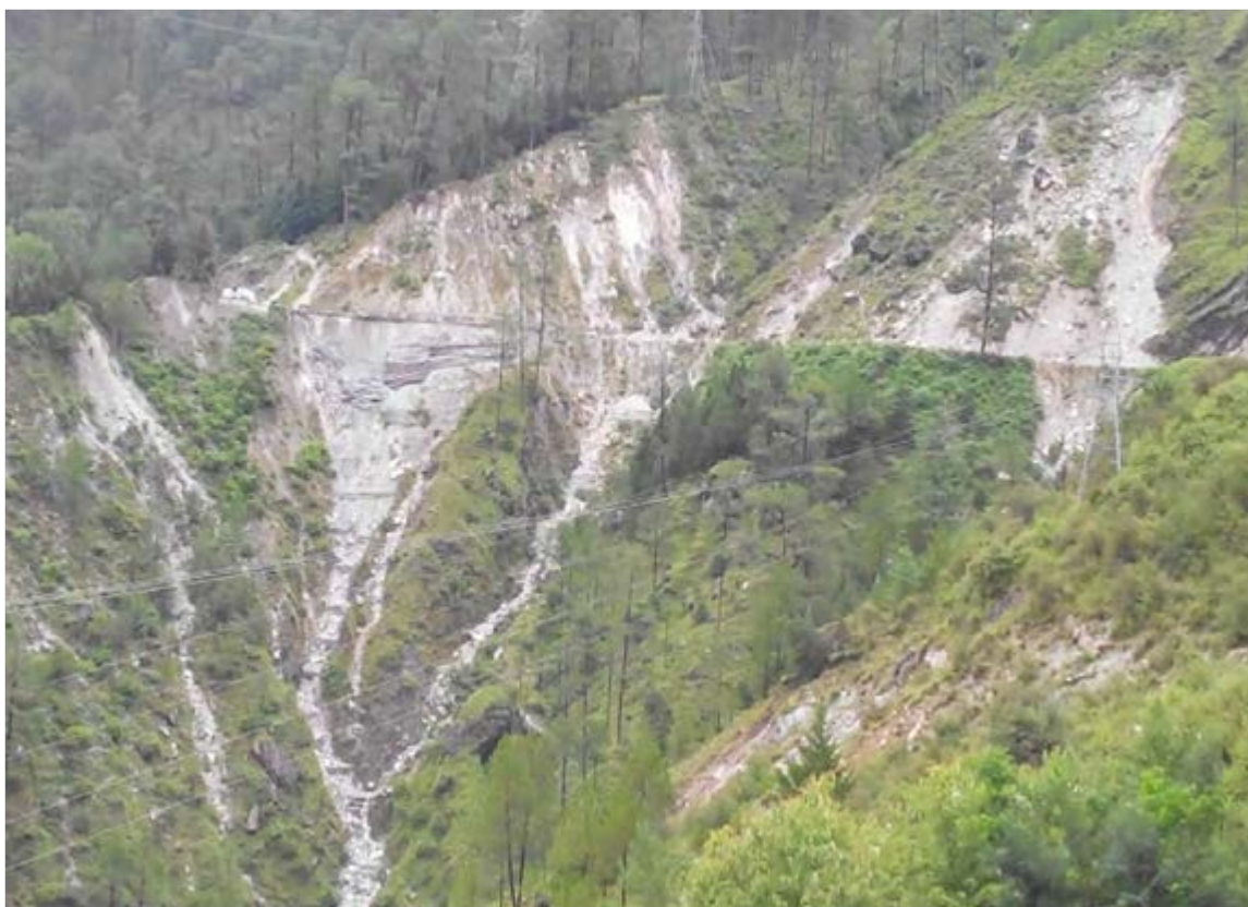
Fig. 1: Panoramic view of landslide
