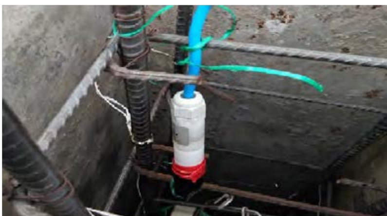
Fig. 2: Placement of embedded permanent reference Ag/AgCl electrode before casting of columns
