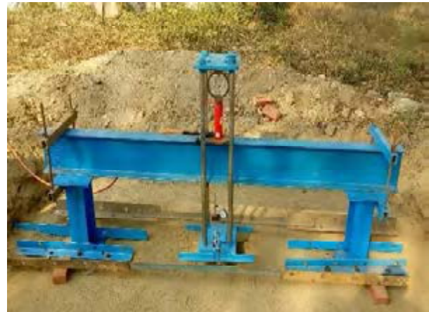
Fig. 5: Pull-out system of openable helical foundation system (in progress)
