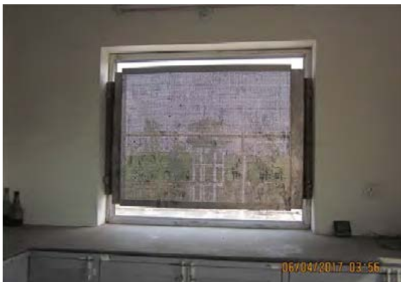
Fig. 1: Solar window with aluminum sheet
