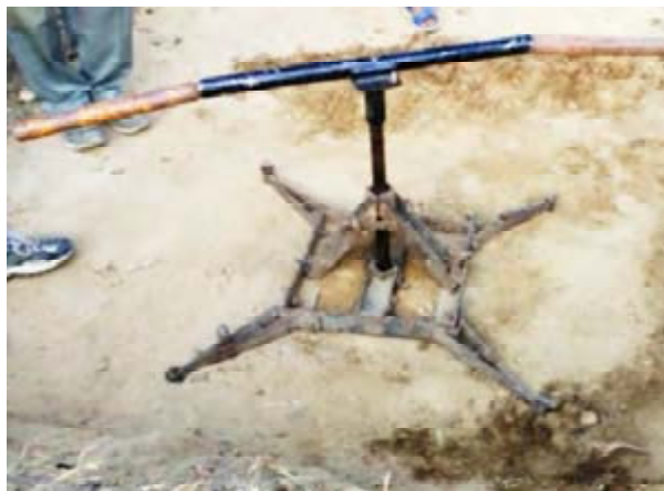
Fig. 4: Installation of openable helical foundation system
