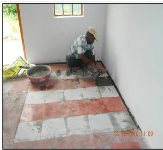
Fig 2: Laying of Tiles in Demo Room
