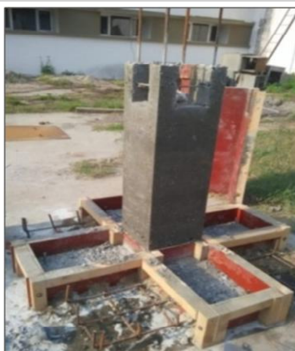
Fig 1: Formwork Preparations & Casting of Precast Pedestal System on Site at Rural Park, CSIR-CBRI, Roorkee
