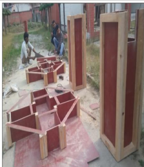
Fig 1: Formwork Preparations & Casting of Precast Pedestal System on Site at Rural Park, CSIR-CBRI, Roorkee
