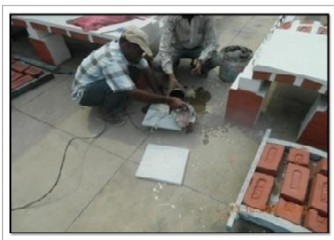
Fig 3: Showing Cutting of Tiles
