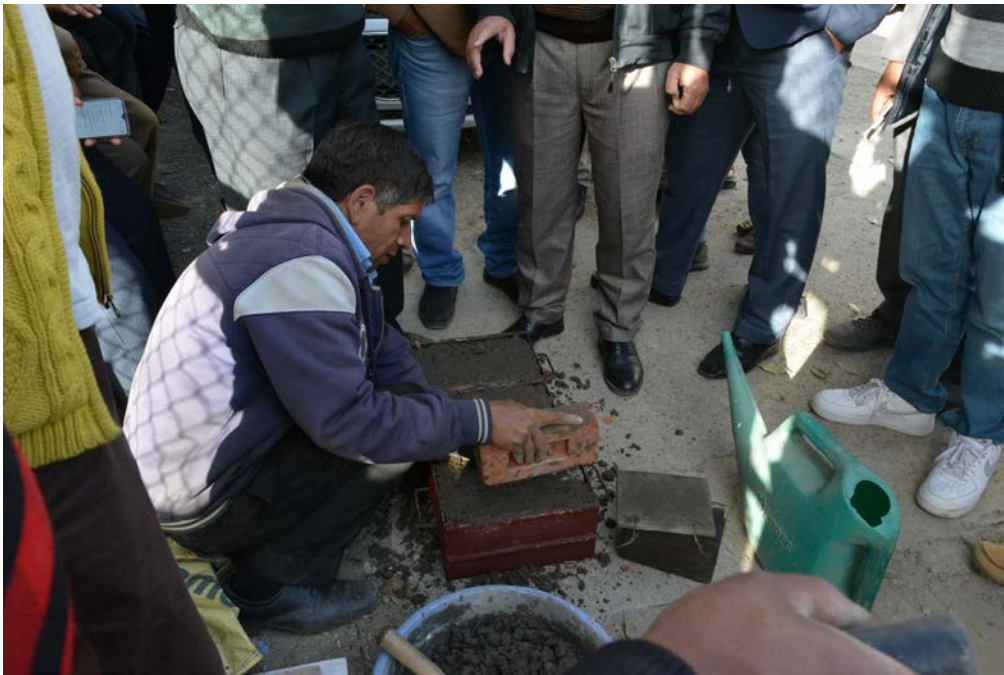
Technical Demonstration of Earthquake Resistant construction practices
