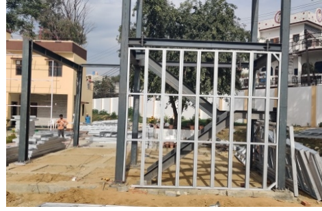
Fig. 2: Erection of CFS Wall Panels
