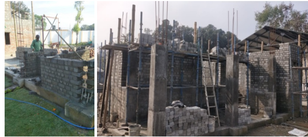
Fig. 3: Construction using Desert Sand Bricks
