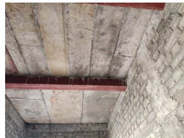
Fig. 5: Placement of Plank & Joist System
