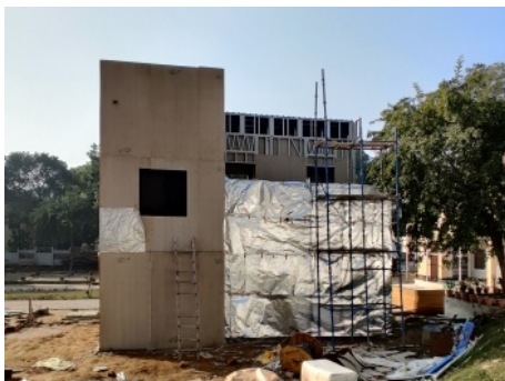
Fig. 6: Second Layer of Sheathing in Progress
