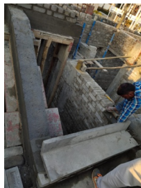
Fig. 4: Placement of Precast Staircases
