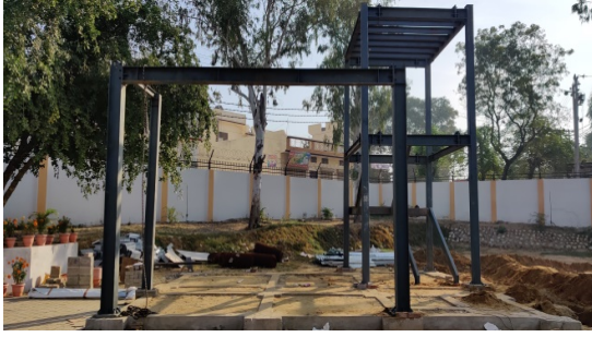
Fig. 1: Erection of HR Steel Columns at Staircase & Front Areas
