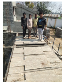
Fig. 5: Placement of Plank & Joist System
