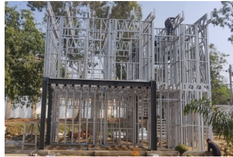
Fig. 3: Erection of First Storey CFS Walls
