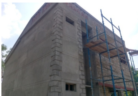
Fig. 4: Plastering Work in Progress
