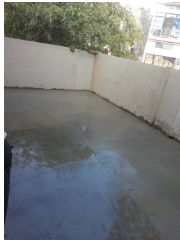
Fig. 4: Casting of First Floor Slab
