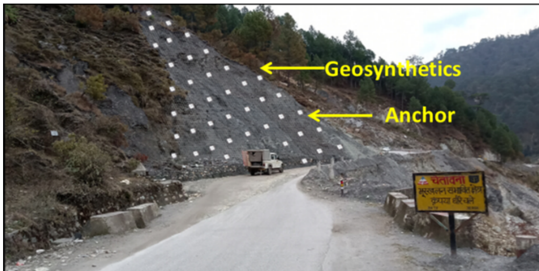
Fig. 8: Proposed Anchored Geosynthetic Reinforcement at Landslide
