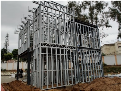
Fig. 3: Erection of First Storey CFS Walls
