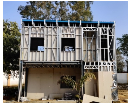
Fig. 5: First Layer of Sheathing Under Progress
