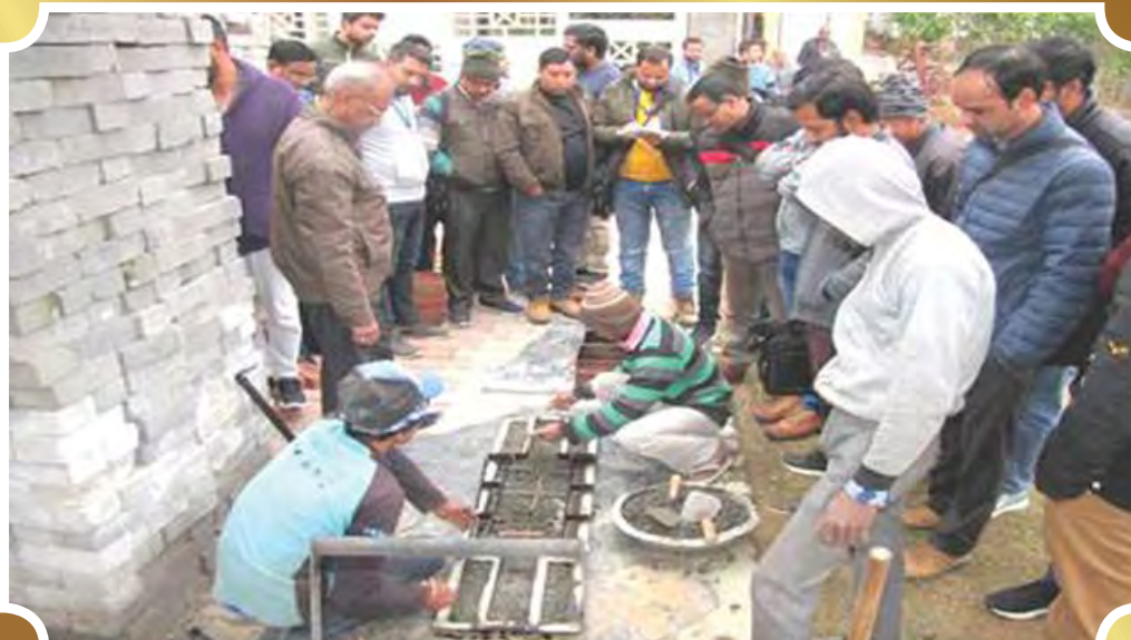
Live Demonstration of casting of Pre-Cast Building Components
