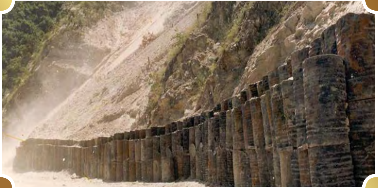
Drum retaining wall for slope stabilization
