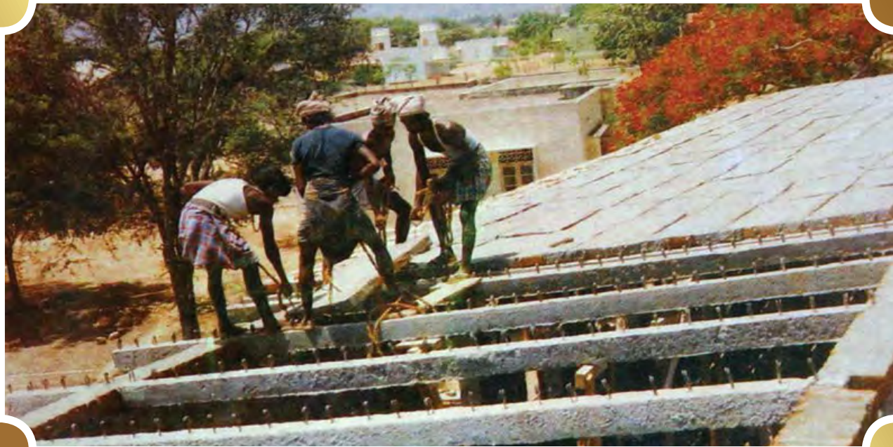
Hostel Building at Gandhigram Rural University (T.N.) using brick panel roofing
