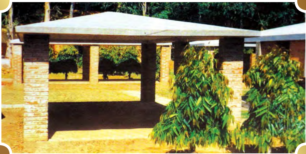
Prototype of unreinforced cement concrete brick roof
