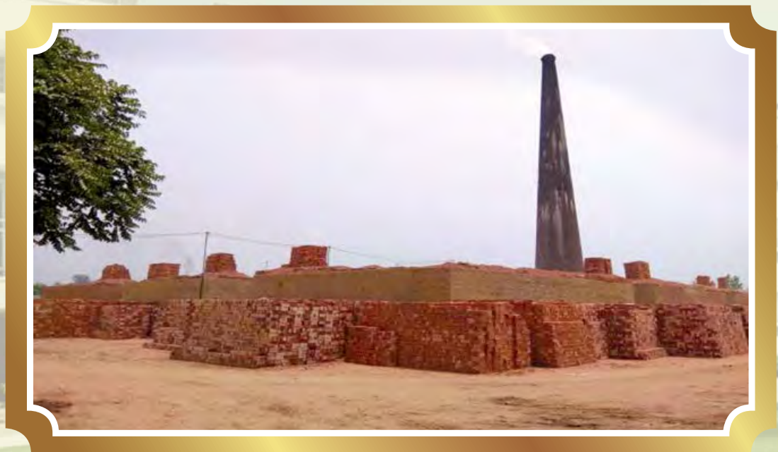
High Draught Zig-Zag Rectangular Brick Kiln
