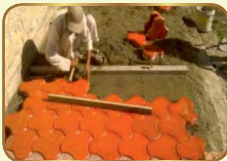
Laying of Paver Blocks
