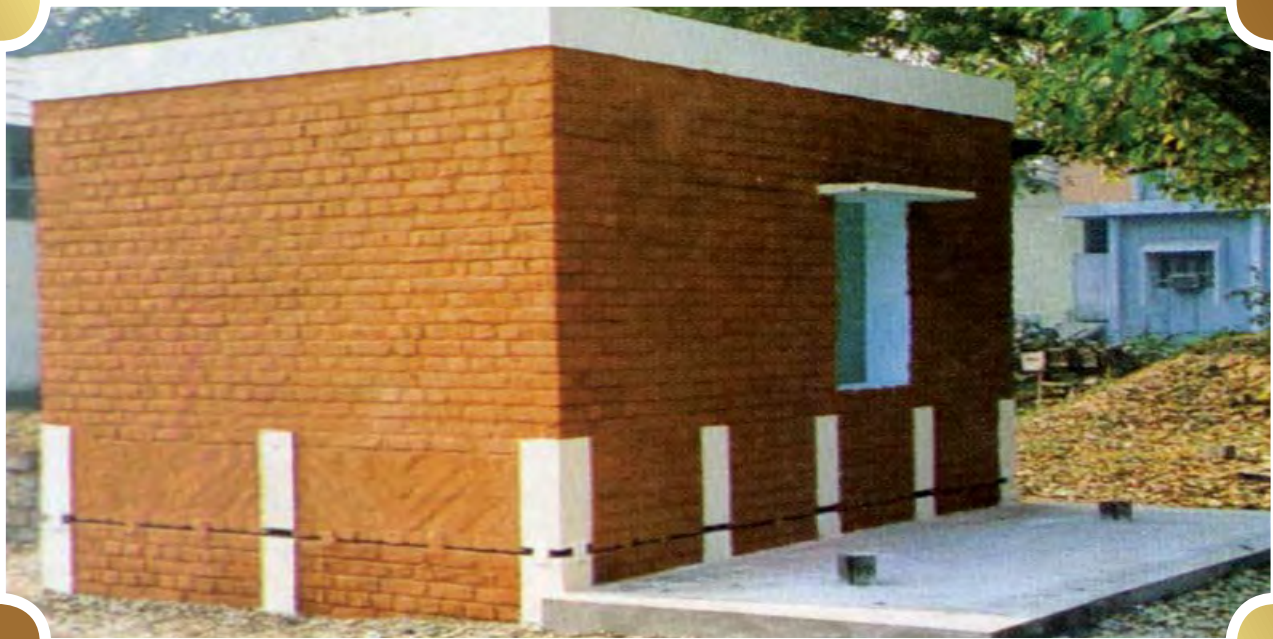
Prototype building with pot panel base isolation bearing
