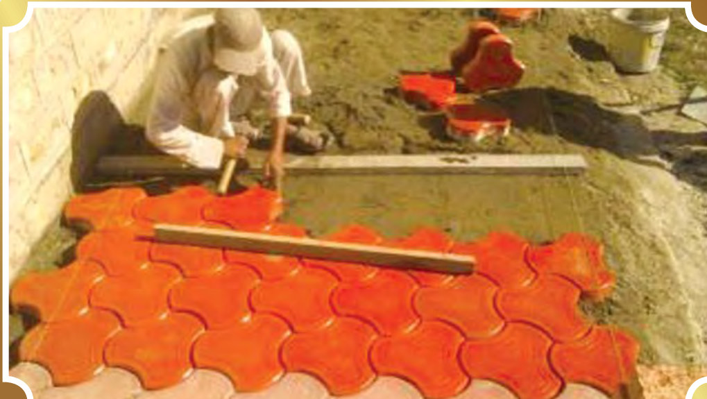
Laying of Paver Blocks
