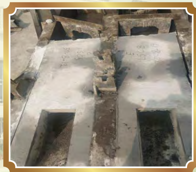
Expa-Mesh Provided in Column
