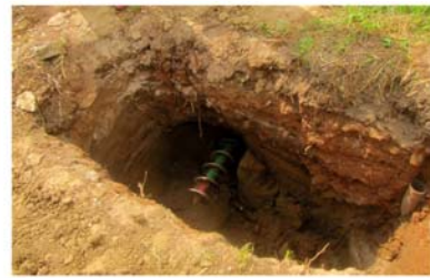
Boring Machine in operation
