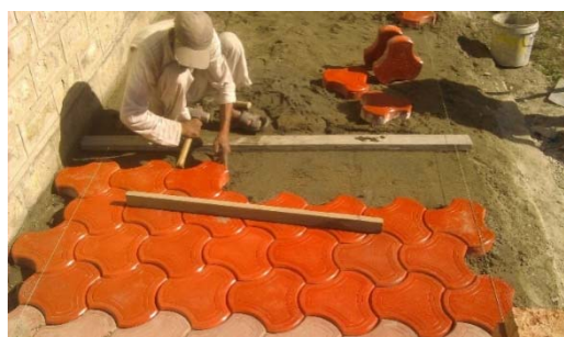
Laying of Paver blocks in CSIR-CBRI
