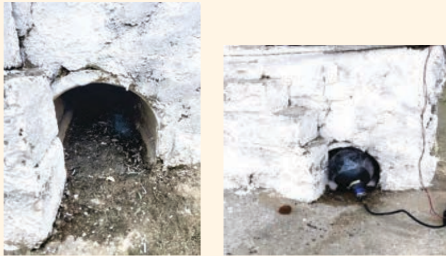
Fig. 5. Retrofitting of 250 mm concrete buried sewer pipe
