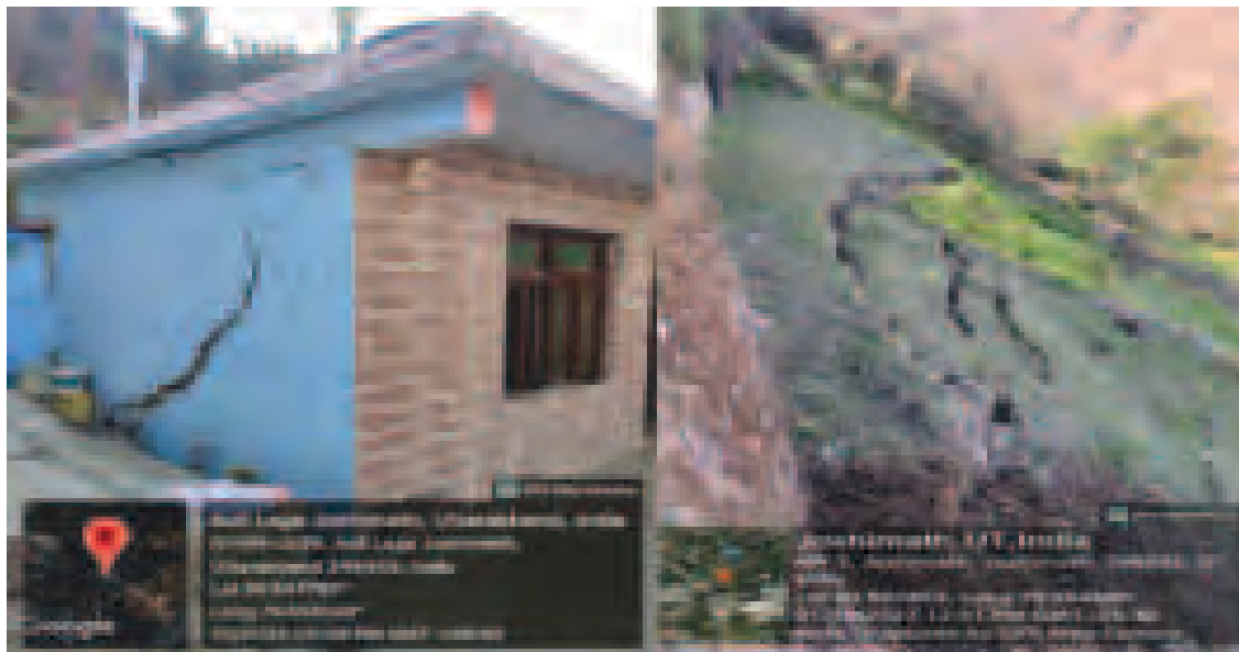
Shear failure towards hill slope
