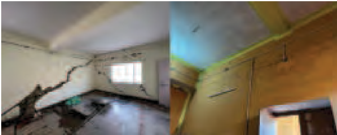
Shear failure due to settlement and rising of floor
