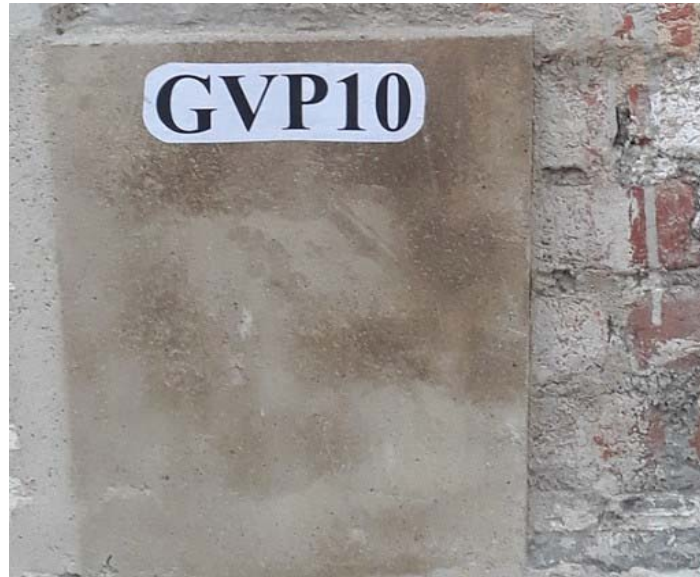
Application of Gypsum Vermiculite Plaster
