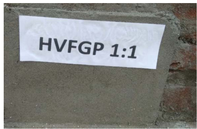
Application of Plaster-sand Mortar (1:1) on Brick Wall
