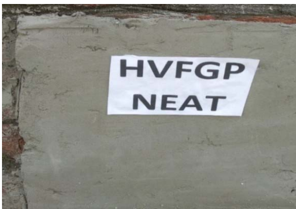
Application of Neat Plaster on Brick Wall
