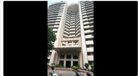
Tower C of Chintels Paradiso, which has been deemed unsafe by experts of CBRI, who conducted the structural audit of the building at Sector-109 near Dwarka Expressway, in Gurugram. (HT PHOTO)
