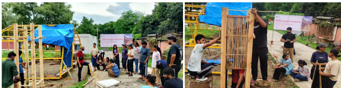
Figure 3. Preparation of Daub by mixing clay, cow dung, straw and sand and pugging
