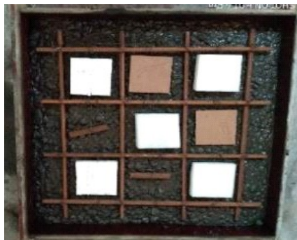
b) Interior of Casted Concrete
