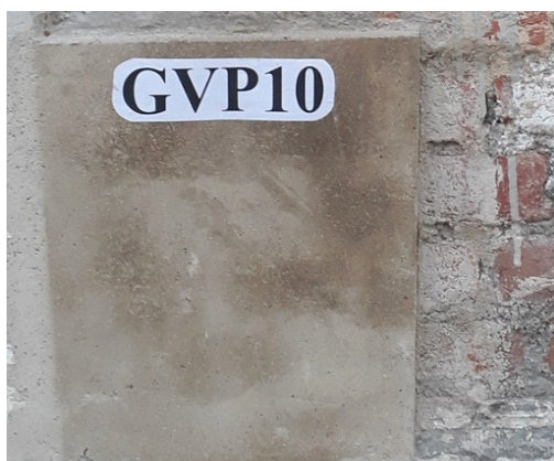
Application of Gypsum Vermiculite Plaster
