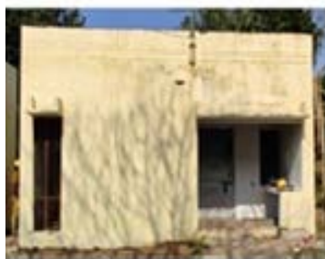
Building front view
