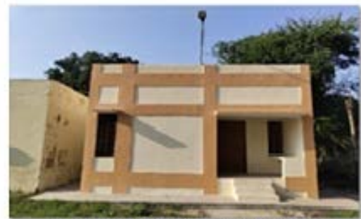
Final View of Strengthened Building
